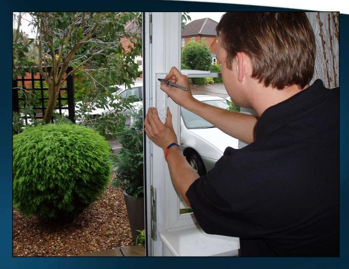
DIS-ASSEMBLE BOXED UNIT AND USE CHASIS TO MARK EIGHT PILOT HOLES AT SHOULDER HEIGHT APPROXIMATELY 1.5m OR 5ft FROM THE GROUND KEEP AWAY FROM LEVER ASSEMBLYS
