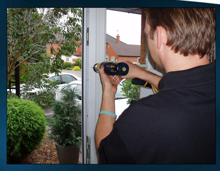
DRILL 1/8 PILOT HOLES ENSURING THE DRILL BIT IS SET SHORT SO NOT TO PASS THROUGH THE FRAME
