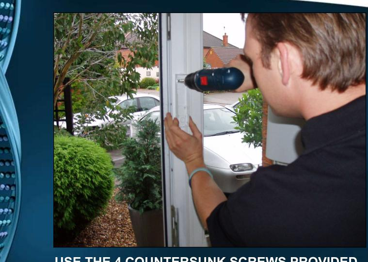
USE THE 4 COUNTERSUNK SCREWS PROVIDED TO SECURLY MOUNT THE CHASIS
